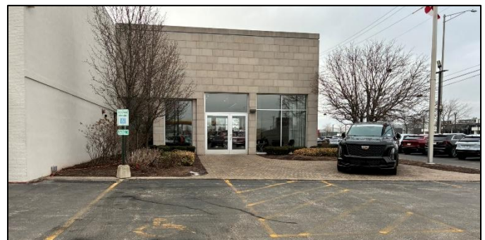
Existing northeast corner of building (where addition is to be located)
